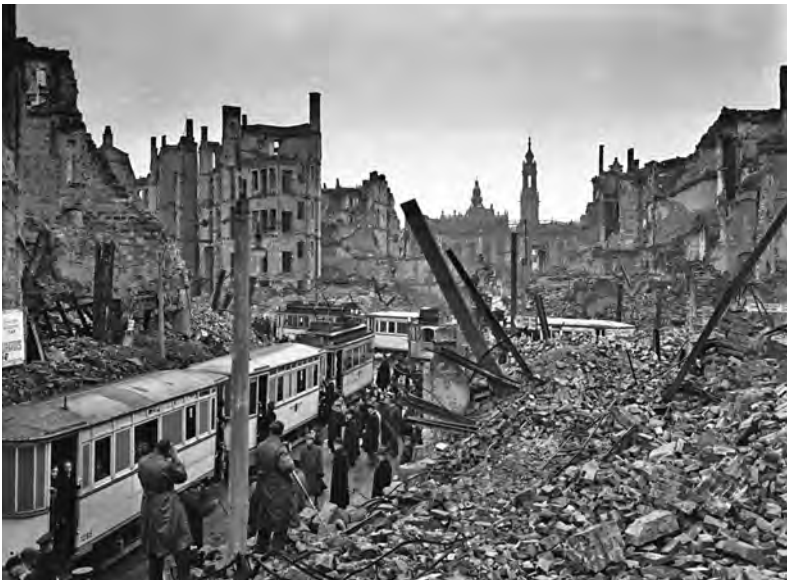
FIGURE 2.14 Dresden, Germany Bomb damage during WWII.
