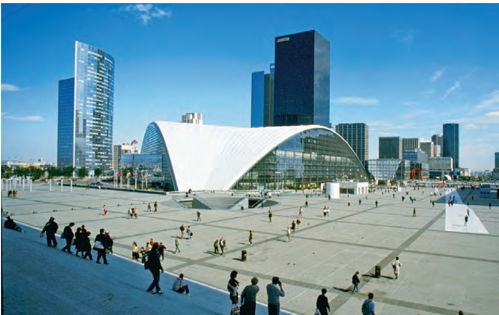
FIGURE 2.39 La Défense One of the largest and most successful growth centers within metropolitan Paris, La Défense was designed by planners to attract office development from the central core of the city.
