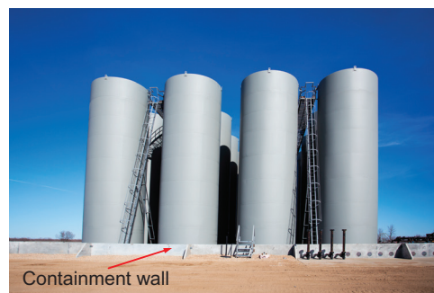
Figure 15.16 Containment wall (also called firewall, bunding, bund wall, or dike).
